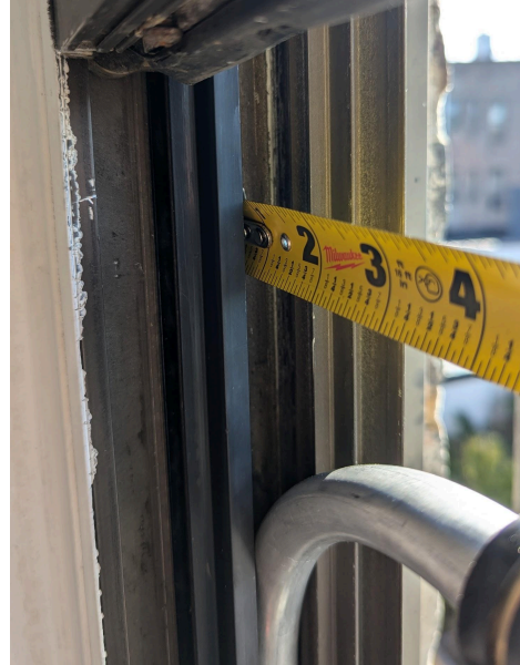
Measure the channel depth.
