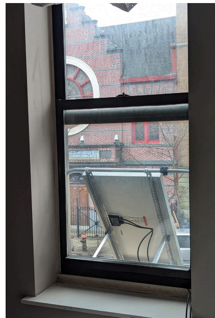
Image: A 50W solar panel mounted in a double-hung window.
